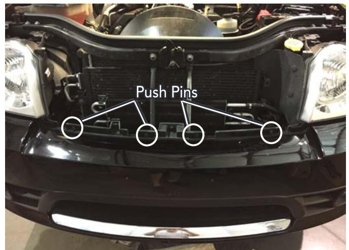
Front Grill Removed
