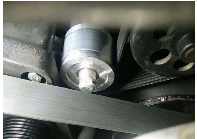
Idler Pulley Installed
