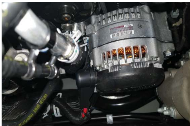
Plastic Cover Installed Over Power Wire
