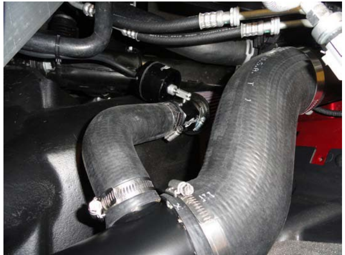
ProFlow Assembly Installed
