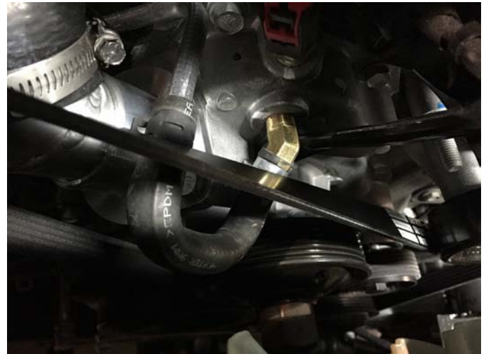
45° Hose Fitting Installed
