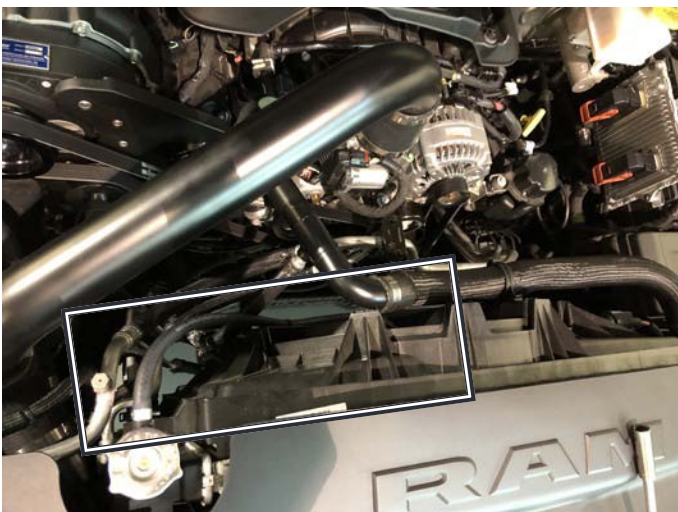
Overflow Hose Installed
