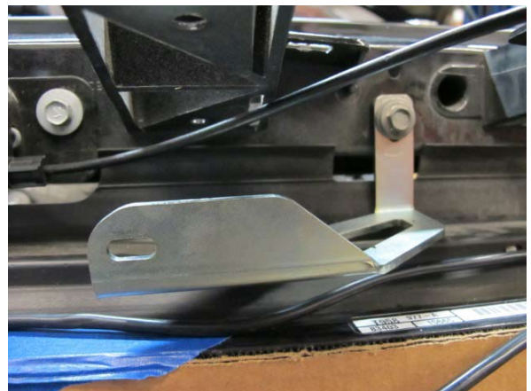
Fig. 6-l: Install upper air/water cooler support bracket
