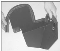
12. Install the provided edge trim onto the heat shield.
